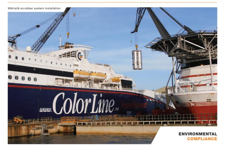
Color Line's high speed ferry 'Superspeed II' sails twice a day between Larvik in Norway and Hirtshals in Denmark with a service speed of 27 knots. Wärtsilä installed four open loop scrubber systems to ensure the ship's full compliance with the International Maritime Organization's (IMO) MARPOL Annex VI regulations, and with EU Directive 2055/33/EC.
