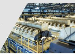
To stay competitive in energy-production markets, power plant operators need to maximise plant efficiency. Introducing higher Miller inlet valve timing and upgrading the turbocharger can reduce specific fuel oil consumption (SFOC), improve reliability and reduce both OPEX costs and emissions. Wärtsilä and ABB have jointly developed a performance upgrade package for W18V46 power plant installations equipped with TPL76C turbochargers.
