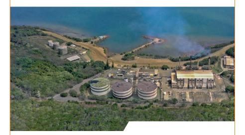
**NEW CALEDONIAN** public utility company ENERCAL wanted to optimise the operational cost and performance of their Nepoui power plant. Before the optimisation project, the fuel consumption of the plant was about 218g/kWh i.e. about 55,000 tons/year.
