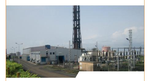
**ENEO CAMEROON'S** Limbe power plant could generate only about 40% of the installed total capacity of 80MW. Wärtsilä's solution was a complete rehabilitation; a total overhaul of four Wärtsilä engines and five alternators. The overhaul covered all critical auxiliaries, including the replacement and upgrade of radiator systems as well as other auxiliaries.
