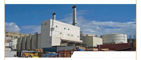
SHANGHAI ELECTRIC POWER, one of the major listed companies of China Power Investment Corporation, reduced both electricity production costs and emission levels at their Delimara 3 Power Plant in Malta. Eight Wärtsilä HFO-fuelled engines were converted to run on natural gas and a new UNIC C3 engine control system was installed.
