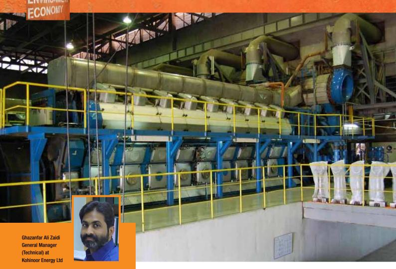
The original turbochargers installed at the Kohinoor power plant in Pakistan had reached their expected service life-cycle. Replacing key components would cause significant costs. Instead of an overhaul, Wärtsilä offered a retrofit solution which would bring higher efficiency and lower fuel oil consumption. A contract was subsequently made to deliver and install eight TPL 76C turbochargers.
