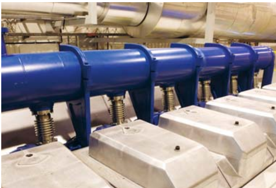
■ Fig. 2 – The large gas common-rail pipe running along the engine.
