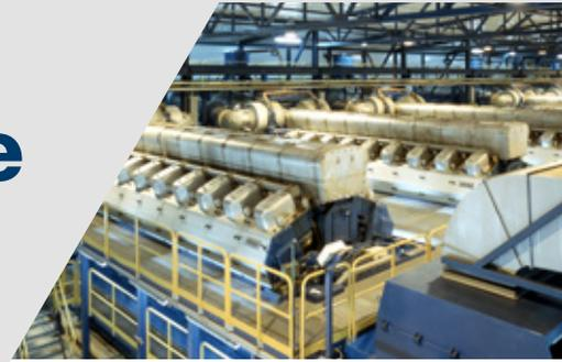
To stay competitive in energy-production markets, power plant operators need to maximise plant efficiency. Introducing higher Miller inlet valve timing and upgrading the turbocharger can reduce specific fuel oil consumption (SFOC), improve reliability and reduce both OPEX costs and emissions. Wärtsilä and ABB have jointly developed a performance upgrade package for W18V46 power plant installations equipped with TPL76C turbochargers.
