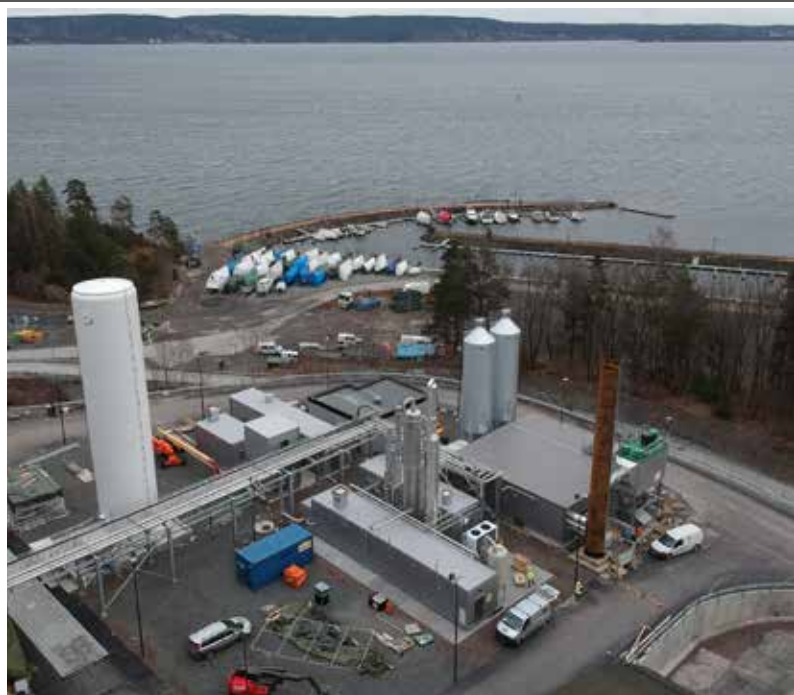
Veas, Norway's largest wastewater treatment plant, fundamental to keep the Oslo fiord clean. It is also an opportunity to produce biogas. The biogas is upgraded and liquefied with Wärtsilä Puregas CA and MR process producing carbon neutral liquid transport fuel for Oslo buses and other heavy transport vehicles
