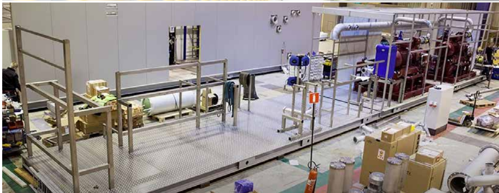
Assembly of process modules in Wärtsilä Kalmar plant
