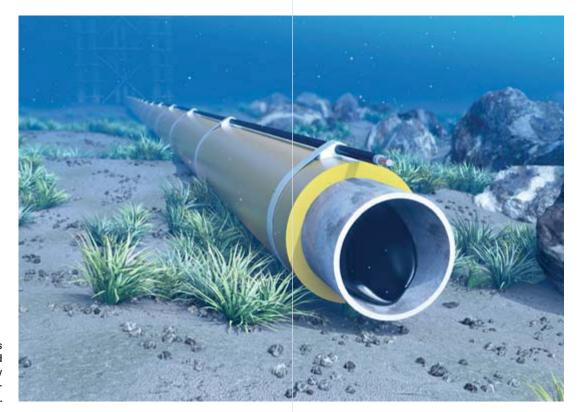
Subsea flow lines face various hazards that may hinder operations or stop them entirely. For instance, water content in the line can form an ice-like structure, known as a hydrate plug, that will interfere with the flow. Another problem common in many regions is the build-up of wax in flow lines.
