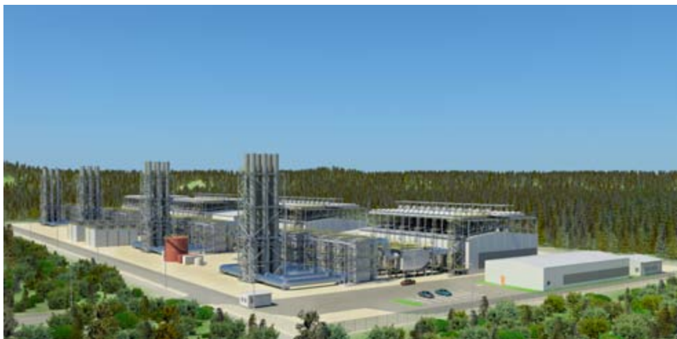
The 500 MW Flexicycle™ power plant based on 24 Wärtsilä 18V50SG units and a steam turbine combined cycle.
