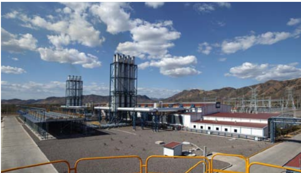
The Lufussa Pavana III base load power plant is located in Honduras and consists of 16 Wärtsilä 18V46 engines having a total output of 273 MWe.
