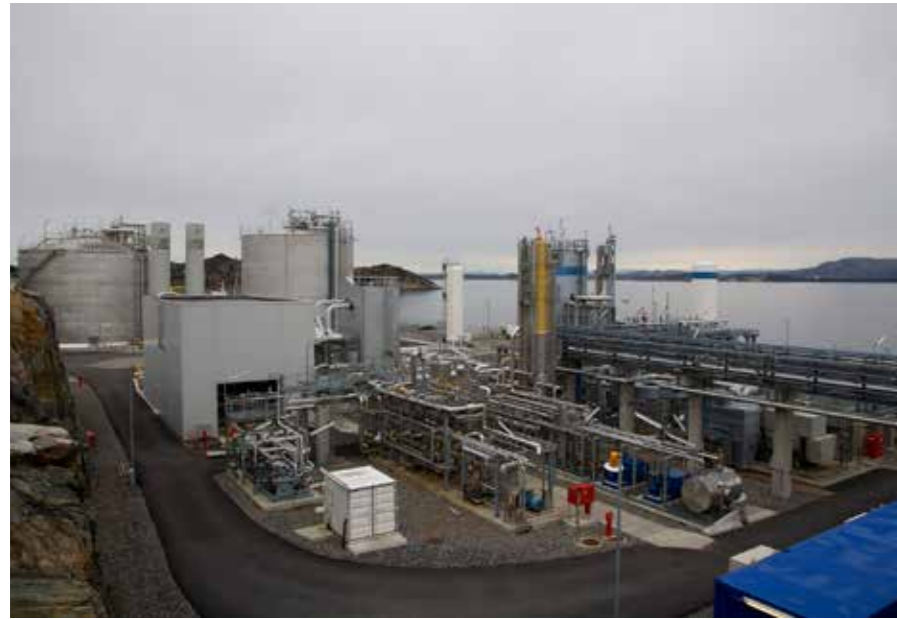
■ Fig. 9 - Kollsnes liquefaction plant in Norway. To the left Kollsnes II, supplied by Wärtsilä, with 84,000 TPA capacity and to the right Kollsnes I with 43,800 TPA capacity. This is an example of a small scale LNG liquefaction plant and export terminal.
