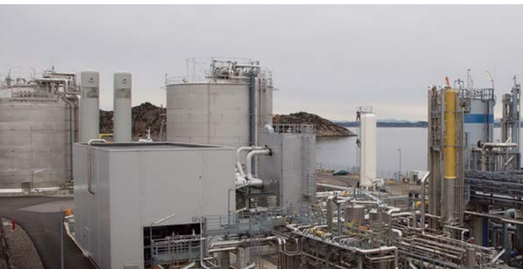
The Kollsnes II plant located near Bergen, Norway features a complete LNG plant including a total gas cleaning system.
