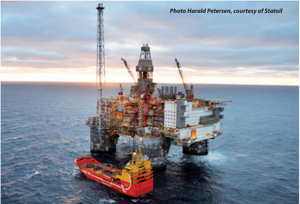
Gravity Base Structure on the Heidrun field
