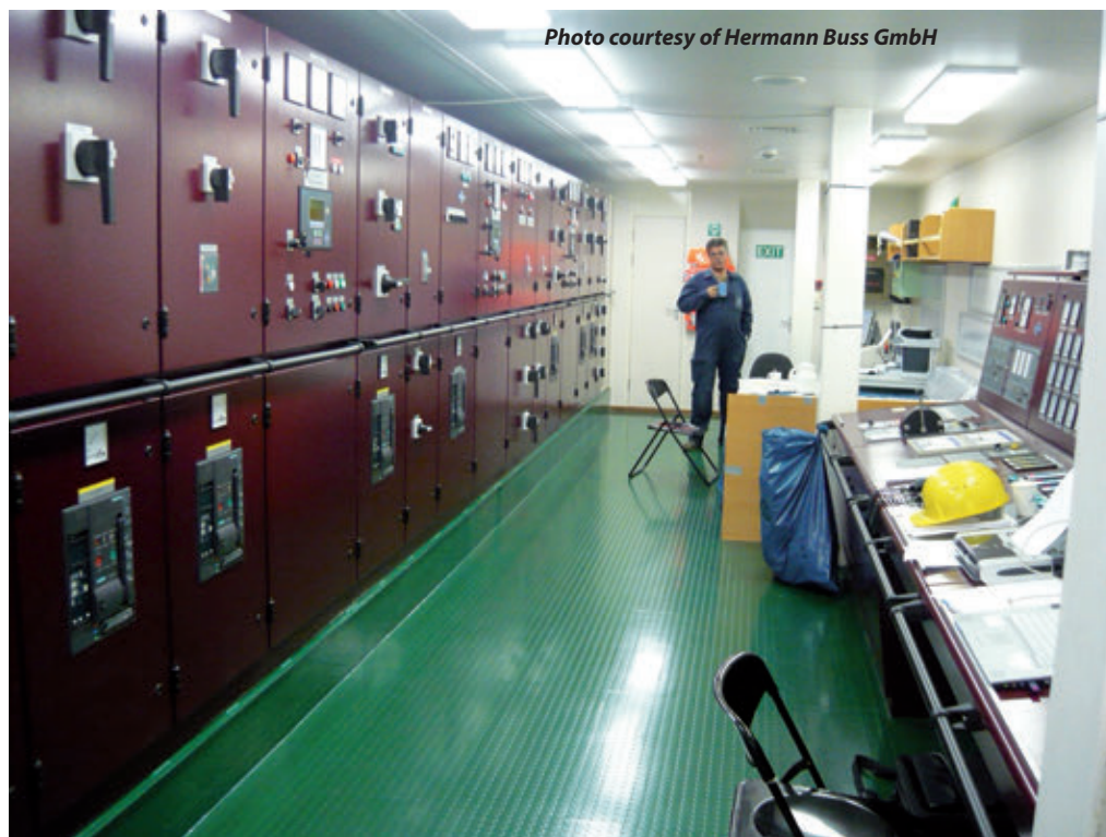
Main switchboard in the Engine Control Room
