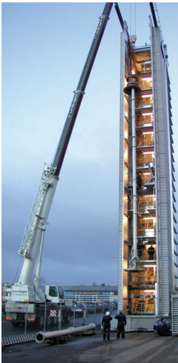
Pump test tower
