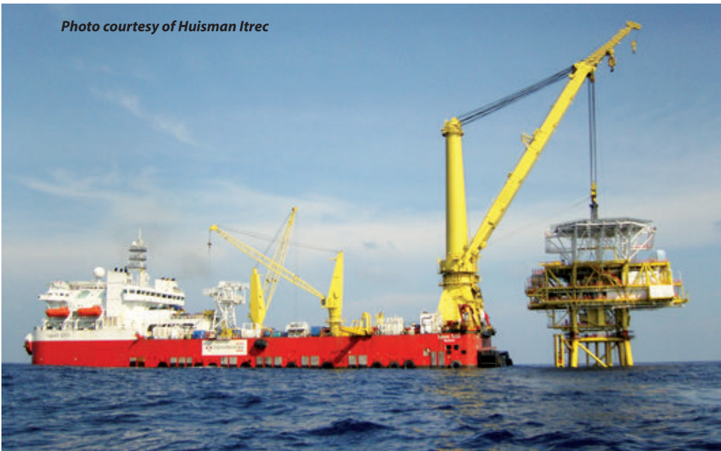
Crane ship SAPURA 3000 placing topside installation
