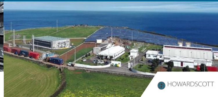
7MW Island Micro grid Recharge AS, Portugal
