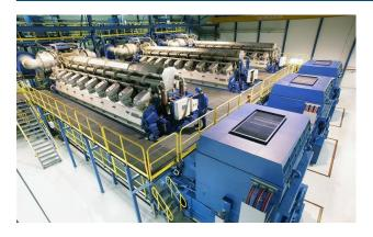
Wärtsilä's technology with fast-starting internal combustion engines will be used to balance the power generation to the grid and ensure system stability
