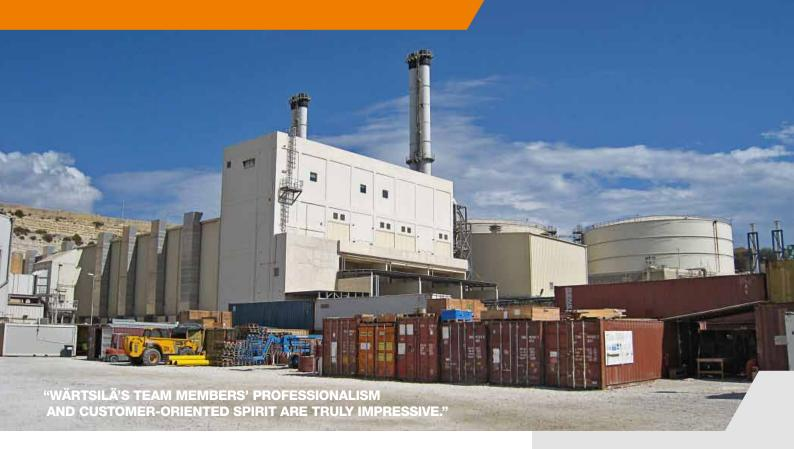
Shanghai Electric Power needed to reduce both electricity production costs and emission levels at their D3 Power Plant in Malta. Eight Wärtsilä HFO-fuelled engines were converted to run on natural gas.
