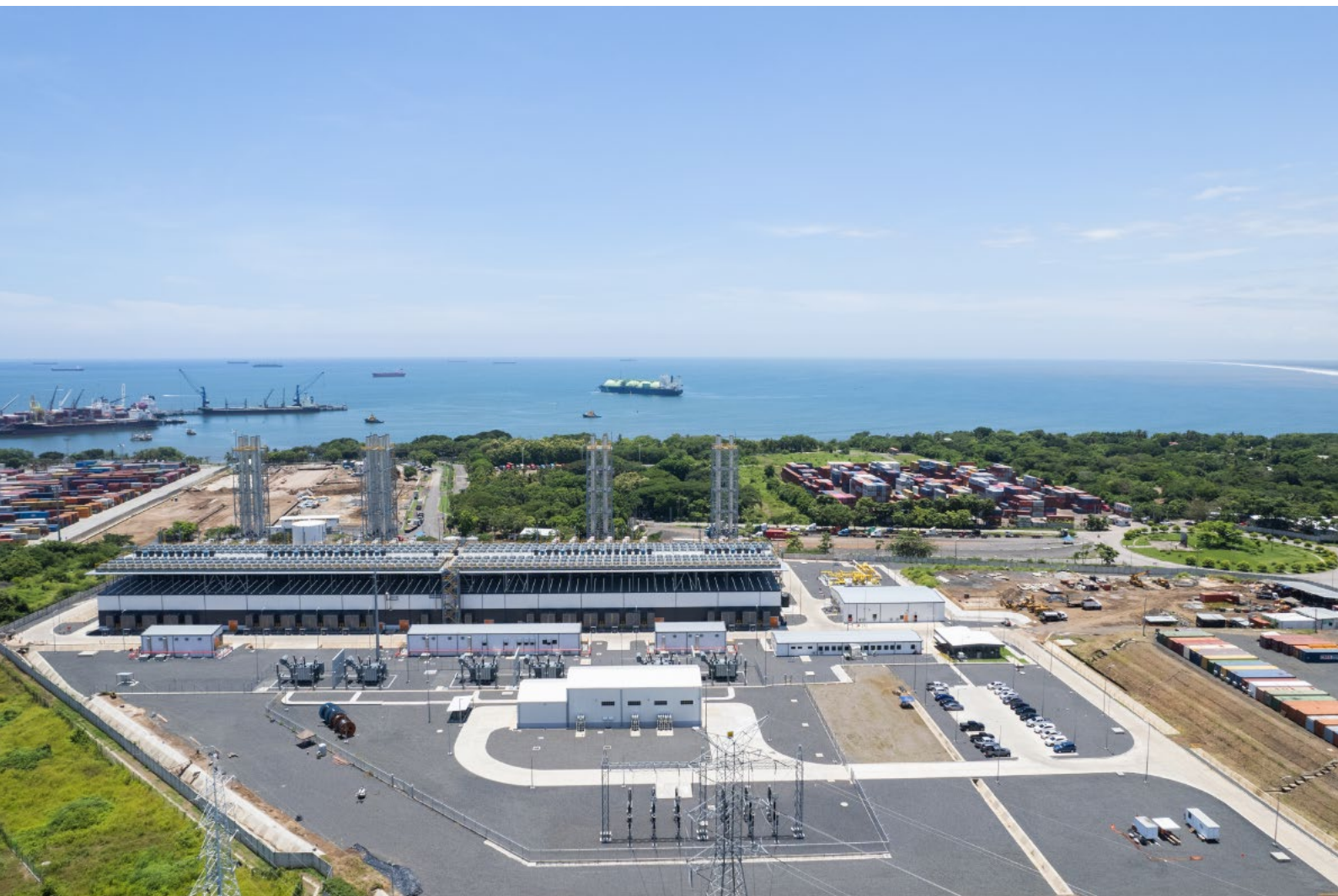
Figure 17: Aerial view of the 378 MW Acajutla Gas Engine Power plant fed directly from the 137,000m 3 FSRU BW Tatiana as seen in the distance.
