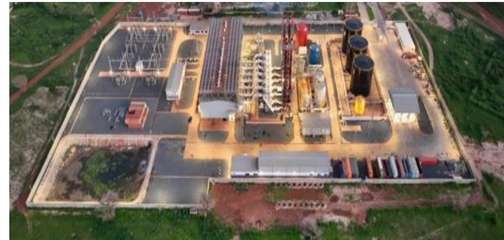
120 MW HFO thermal power plant convertible to gas
