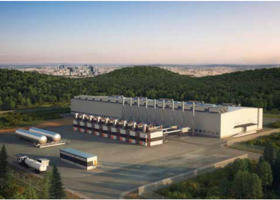
A site with five Wärtsilä Modular Block Compact units, each with a Wärtsilä 12V34SG engine. All units are connected and share their middle walls but remain functionally independent. The stand-alone building in the lower-right corner is a medium voltage switchgear building used as a point of interconnection between the generating sets and the public power grid.
