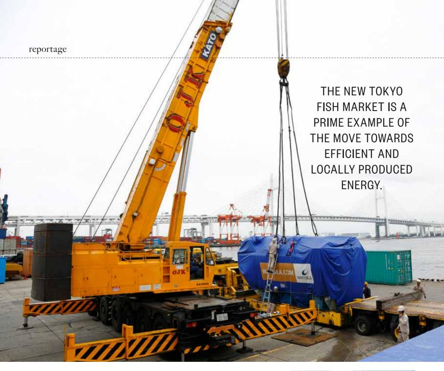
At the dock, the power Plant's new giant engine is hoisted onto the transport truck. Securing it for the journey is critical.
