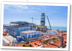
The new Cap des Biches power plant that was inaugurated in Senegal in June proceeded from concept to live generation of electricity in just 14 months. The 53 MW Flexicycle plant comprises three Wärtsilä 46 internal combustion engines and a combined cycle heat recovery system. The power plant will feed electricity to the national grid under a 20-year power purchase agreement (PPA) between ContourGlobal and Senelec, the national electricity company of Senegal.
