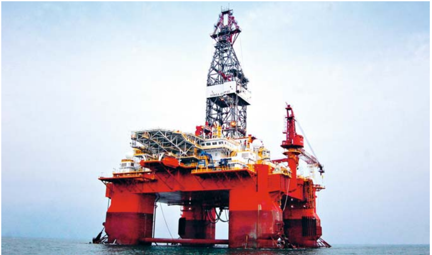
■ Fig. 1 – A Propulsion Condition Monitoring Service system will soon be installed on the eight steerable thrusters of the Songa Eclipse, one of the mobile offshore drilling units owned by Songa Offshore. The Eclipse sails under ABS class society guidelines.
