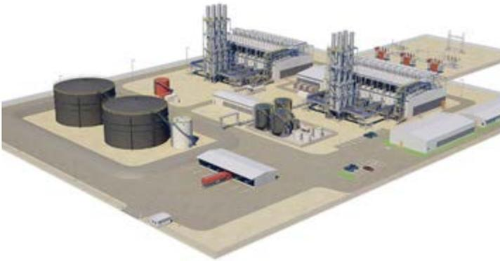
Fig. 12 – A typical onshore power plant layout.
