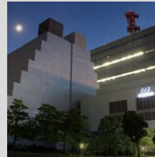
Combined heat & power plants (CHP)
