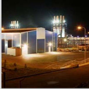
Flexible base-load power generation
