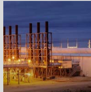
Flexible grid stability power plants
