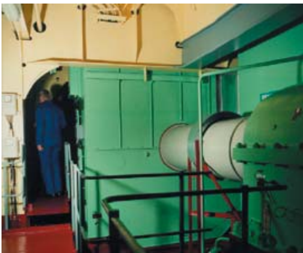
Fig. 8: Typical shaft motor/alternator of about 6MWe output installed on the intermediate shaft of a large container ship. (Siemens) [04#044]
