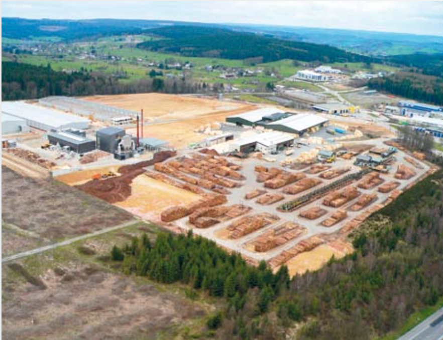
Fig. 1 – The second Wartsilä bio-fuelled power plant ordered by Renogen will be situated right next to the existing, identical plant in Amel, Belgium.
