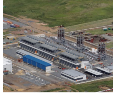
10.7. The largest power plant running exclusively on natural gas engines on the African continent, in Sasolburg, South Africa, was inaugurated.
