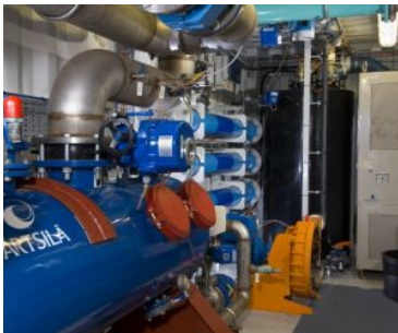
16.5. Wärtsilä AQUARIUS EC Ballast Water Management System received the IMO Final Approval status.
