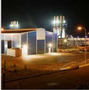
Flexible base-load power generation
