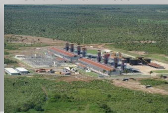
Geramar I & II – 330MW
