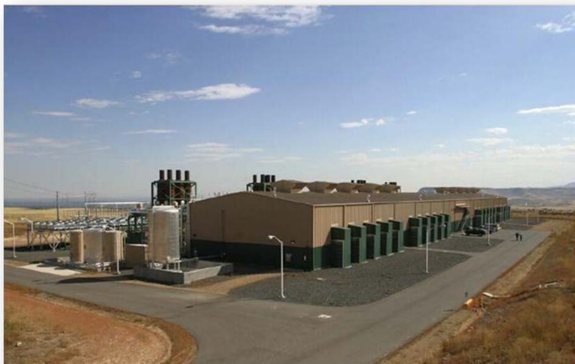
Dispatcher's dream plant Plains End 227 MW Colorado
