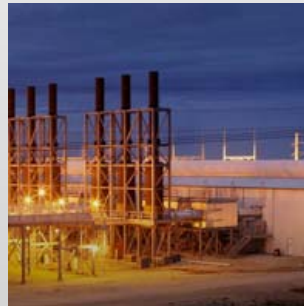
Flexible grid stability power plants
