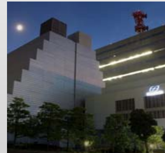
Combined heat & power plants (CHP)
