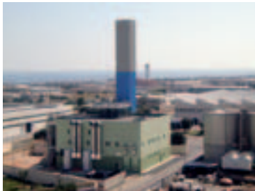
The Pentesilea plant (16 MW) in Italy is fired using bio-oil, such as palm oil.
