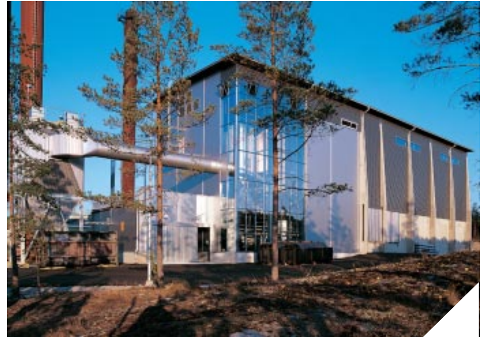
Tammisaaren Energia Oy, Finland, 15 MWth.
