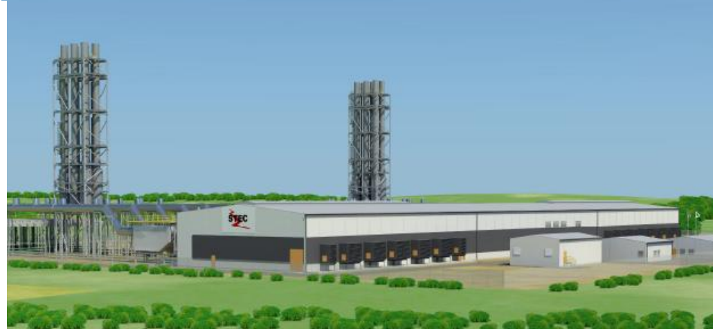
Rendering of STEC's new Red Gate Power Plant: 12 x Wärtsilä 18V50SG, 225 MW
